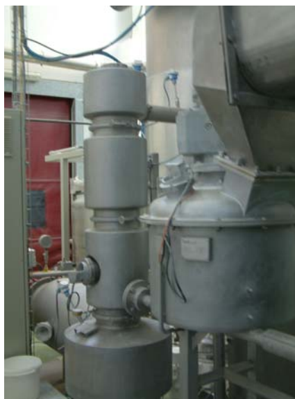
At present. Feed tank and drying chamber
